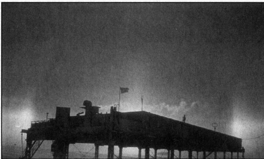
This is a photo of the Accommodation Building at Halley Base, Antarctica. The legs of the building need to constantly be jacked up to keep the building above the rising snow level. The amateur radio station is located in a smaller but similar building known as the Space Science Building, or SSB—an apt place to be. In this view you can see the sun's rays forming a mystical effect around the building.
